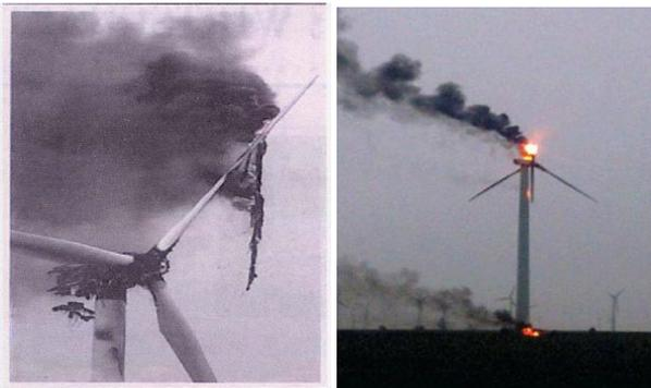
Fig 1. Wind turbines exposed to lightning strokes
